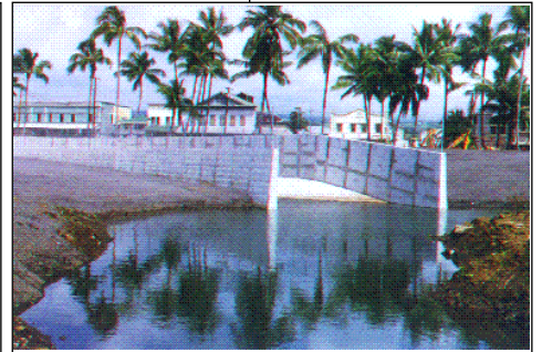
(Left) Lt. Col. Graves listens while Hilo resident Harold Desaki recalls past thunderstorms that flooded Hilo. (Right) At the downstream limit of the channel, future floodwaters will flow into the Waiolama Canal and be dissipated. Buildings in downtown Hilo appear in the background.
